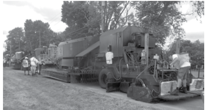
At work resurfacing
